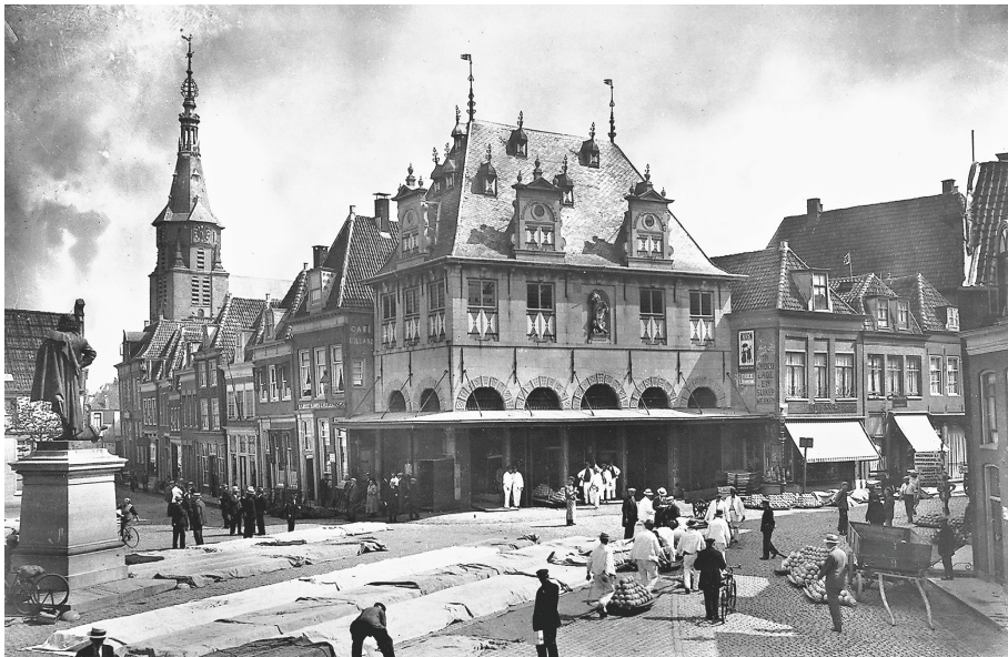
63 Hoorn weigh house from the southwest, photograph before 1930
