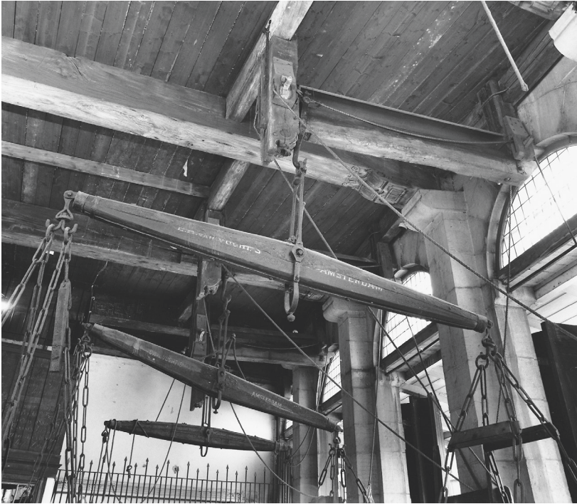
95 Hoorn weigh house, ceiling detail with the trolleys and scales, photograph 1982
