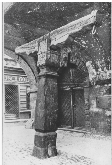
98 Vertical wooden scale below the arch of the so-called weigh house in Silesian Nysa (formerly Neisse)
